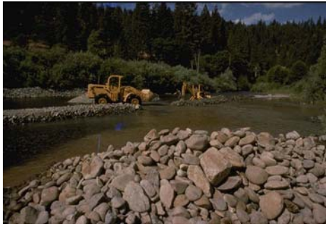
Figure 9.5: Heavy equipment. Avoid heavy equipment in stream channels unless absolutely necessary.
