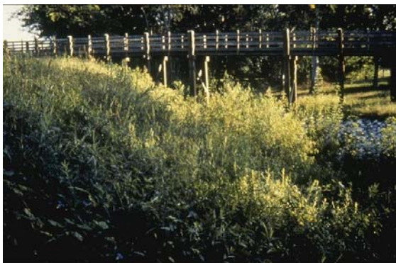
Figure 9.20: Remedial maintenance. Soil bio-engineering used to repair failing revetment.
