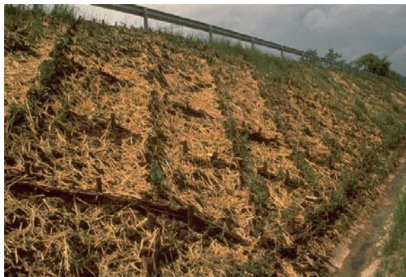
Figure 9.13: A well-mulched site. Mulching is an effective method for improving the final outcome of stream corridor restoration.
