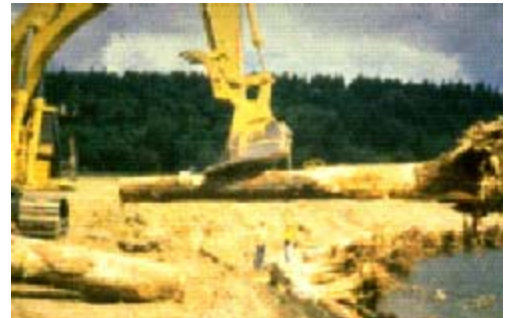
Figure 8.43: Installation of logs with intact root wads. An advantage to using tree revetments is the creation of habitat for invertebrates and fish along the streambank.
