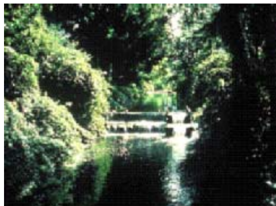
Figure 8.28: Grade control structure. Control measures can double as habitat restoration devices and aesthetic features.
