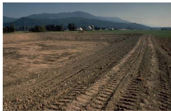
Figure 9.11: Track-roughened area. Rough-textured slopes provide a much better environment for seedlings than do smooth-packed surfaces.
