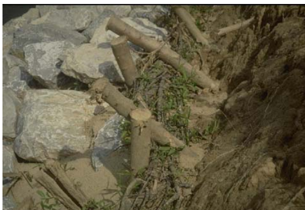
Figure 8.12: Revegetation with the use of deeply planted live cuttings. In arid regions, poles or cuttings of species that sprout readily are often planted to depths that assure contact with moist soil.
