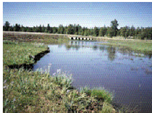
Figure 4.20: Multiple elevated culvert array at crossing of wet meadow. (June 1997.) The culvert spreads flow and decreases erosion energy, captures sediment upstream, reduces flood peaks, and prolongs baseflows.
