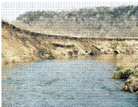
Figure 7.23: Bank instability. Determining if instability is localized or systemwide is imperative to establish a correct path of action.
