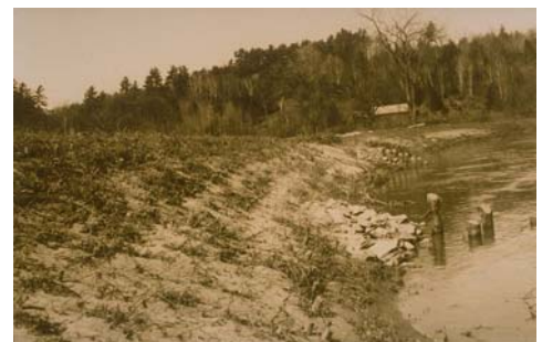
Figure 6.12: Brushmattress and plantings after spring runoff in March 1938. Note pole jetties. Brush-matting involves applying a layer of brush fastened down with live stakes and wire.
