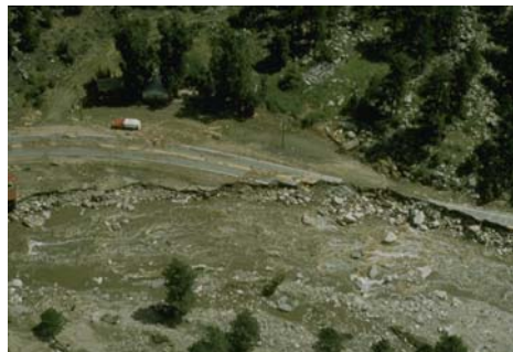
Figure 4.12: Bank erosion. The cause(s) of bank erosion should be identified.
