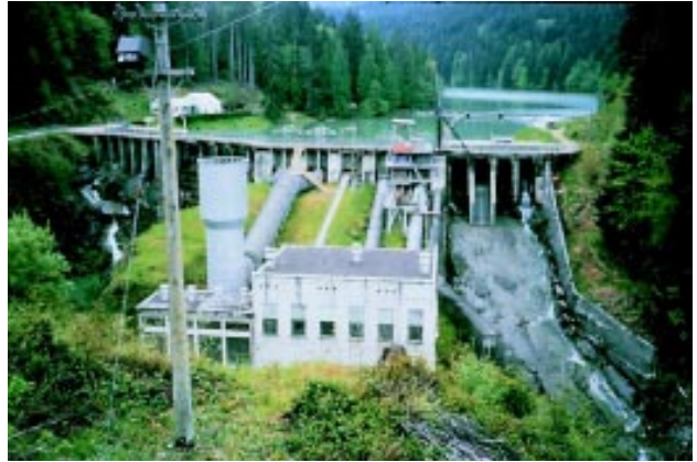
Figure 5.8: Elwha Dam. Fish passages were not constructed when the dam was built in 1910-1913.
